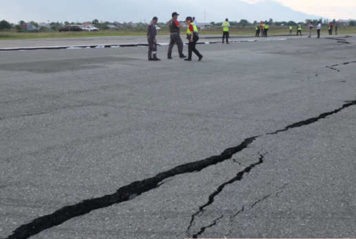
Ground Cracking at Palu Airport
